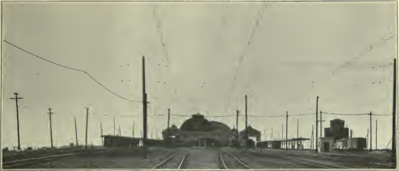
FIG. 525. OVERHEAD CONTACT SYSTEMS. Catenary Construction, 1,200-Volt Direct Current Terminal Yard, Southern Pacific Railroad, Oakland, Cal.
